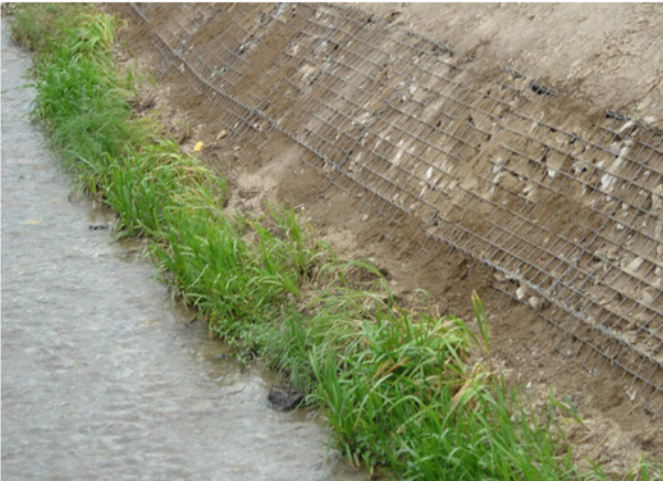
unrolled along the waters edge and fixed on the gabion mattresses
