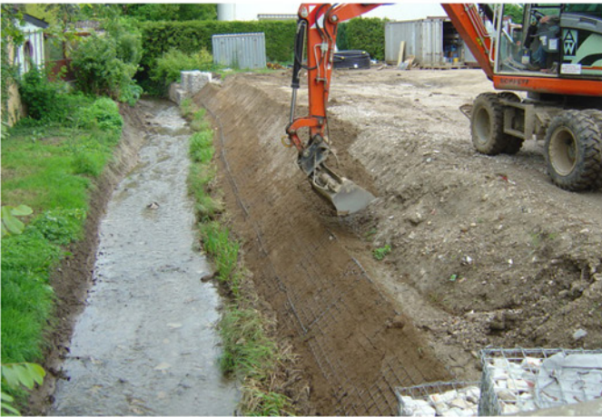
Onsite works in spring 2004; the slope are being covered with soil.
