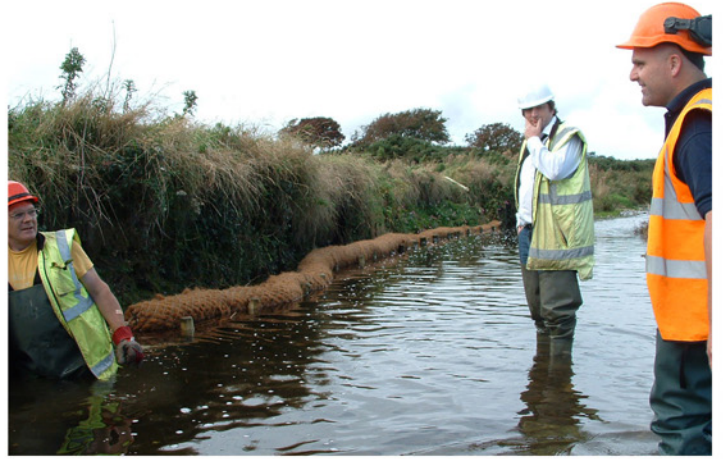
Above: Salix supervision and on site training of works
