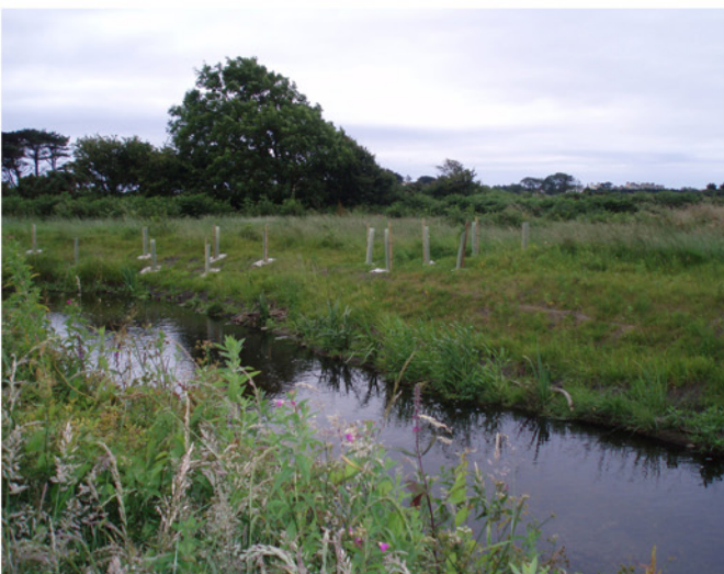
Above : The bioengineering solution after 6 months growth
