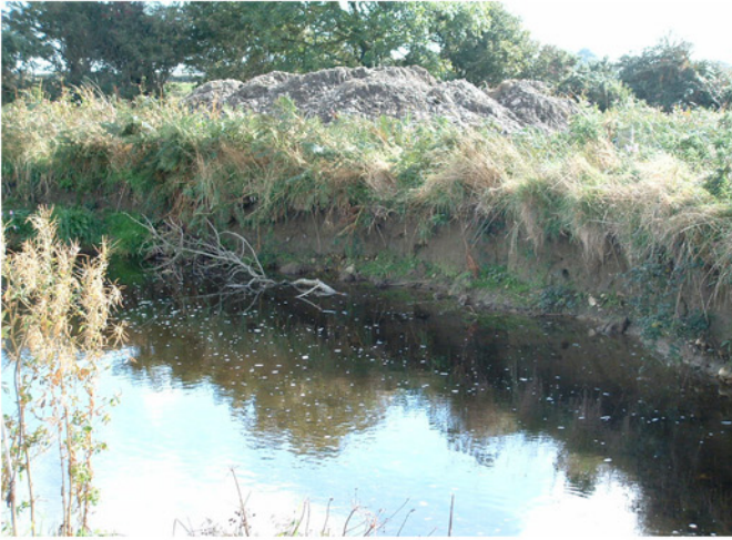
Above: Rock Roll installation at the toe of the bank
