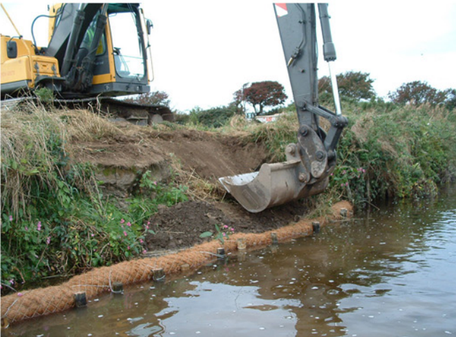
Below: The river bank is graded and infilled
