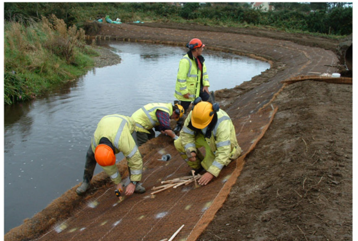
Below: Installation of the C350 erosion control geomat
