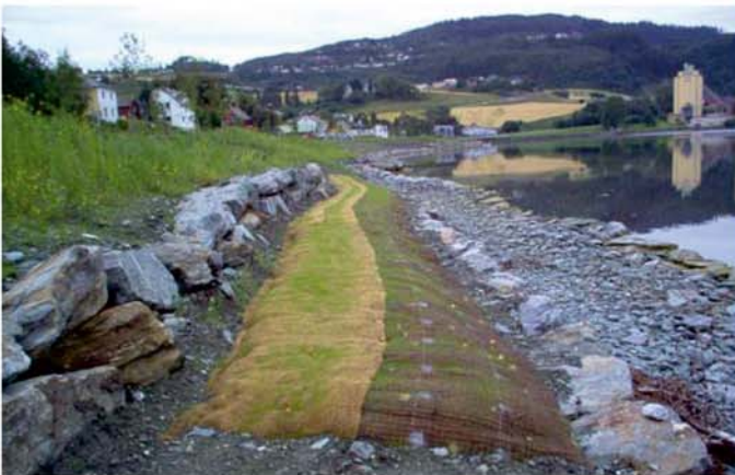
Just after installation
