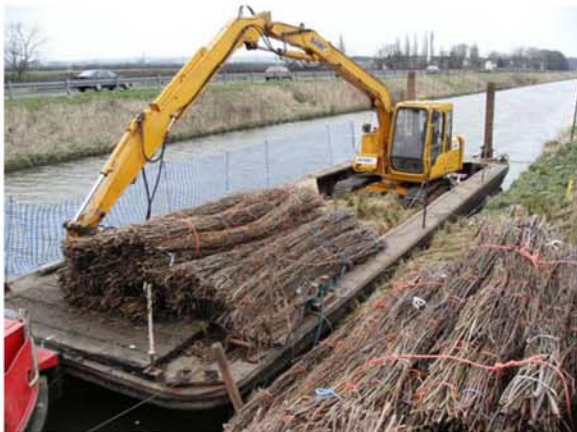
Above Left : Erosion on the Foss Below : Brushwood fascines
