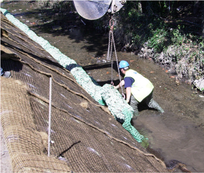
Above: Rock Roll installation at the toe of the bank
