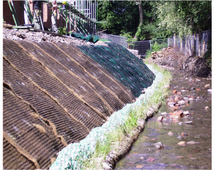
Above: The completed bioengineering solution.
