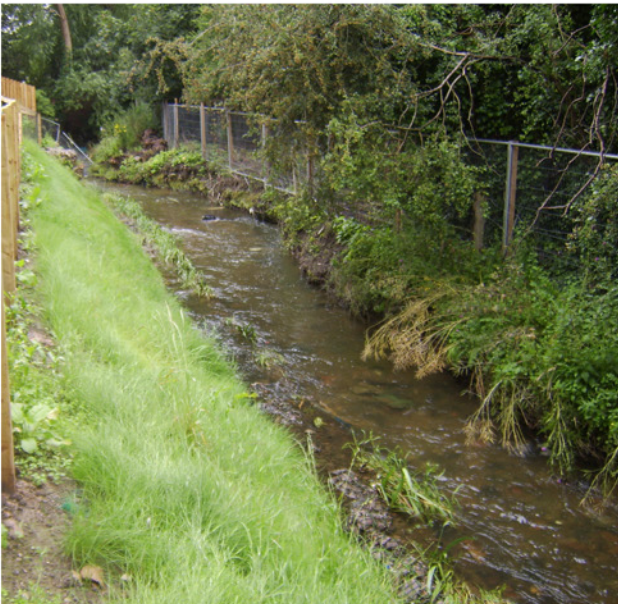
Above: The bioengineering solution 8 weeks after installation, after a major flood event.
