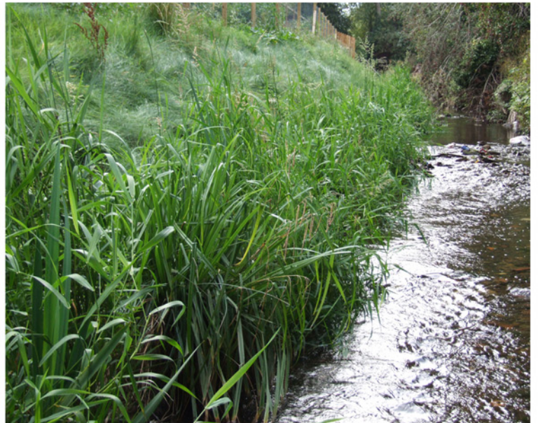
Above: The bioengineering solution 4 months after completion
