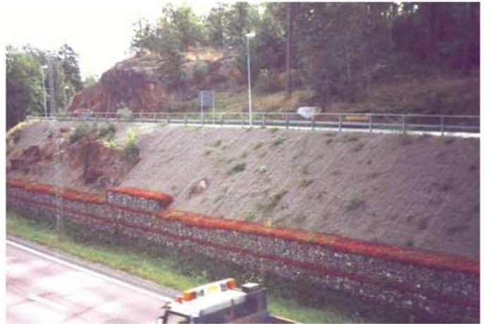
Gabions and coir geotextiles
