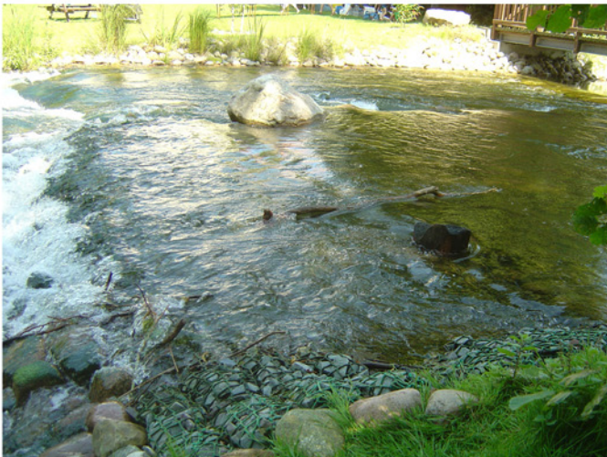
Rock mattresses have been applied to reinforce the spillway.
