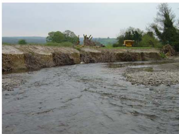
Above : Tree Root Revetment After Installation
