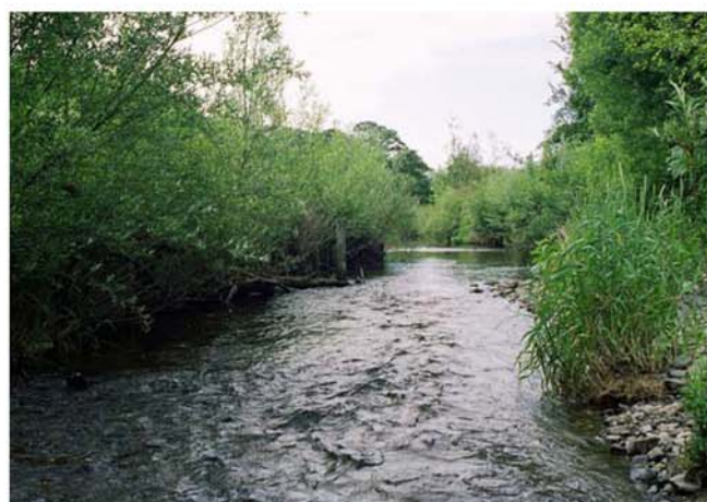
Live Willow fascines and bank grading 2 years after
