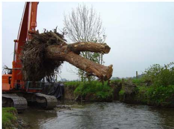
Above : Tree Root Revetment Being Installed
