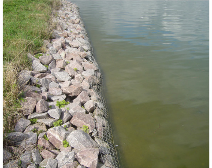
Above: Initial "hard" revetment solution.
